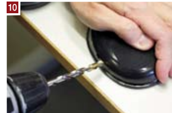
Drilling and routing of the wire (HGU-55 and ACS style)
